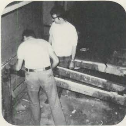
Lance Johnson and Dave Knudtson at the Fargo Theatre, remove pit floor. (S. Carlson Photo)
