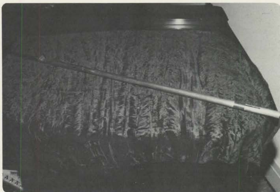
Single pipe repaired.
