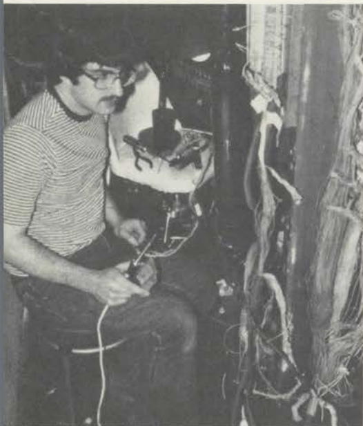
Extensive revamping of the relay and switches was a tedious job for Tom Delay.
