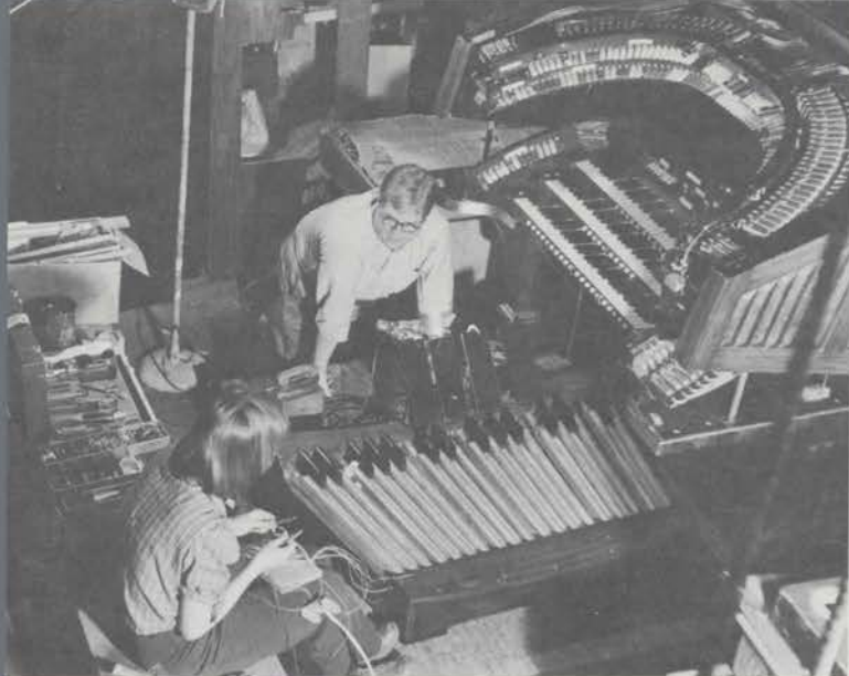
Organ technicians Dolores Rhoads and Jim Roseveare check electrical connections on the Oakland Paramount's huge four-manual Wurlitzer organ console. Solid state equipment will transmit impulses from each key, tab and pedal on the console to the multitude of devices which control the instrument's pipes, percussions and special effects.
