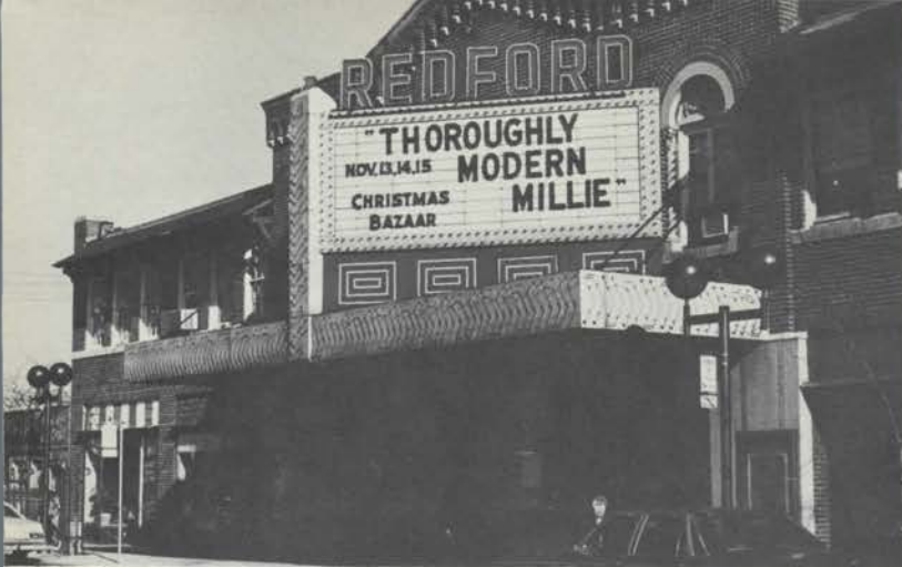
A bimonthly movie series continues to provide a steady source of revenue. The present marquee is an adaptation of the original.
