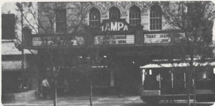
The Tampa Theatre, home of the 3/12 Wurlitzer being installed.
