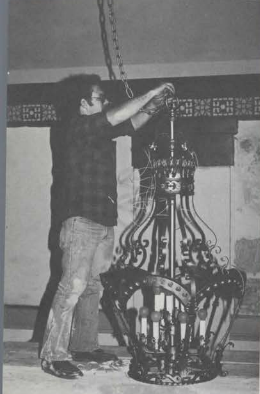
Dave Vincent attaches the support chain to the fixture. The time has finally arrived when it may be nudged off the scaffold.
