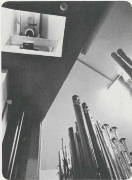
View of the bottom of a tremulant, upper left, located in the tremulant room in Solo Chamber. Tremulant rooms were built in each chamber to eliminate noise.
