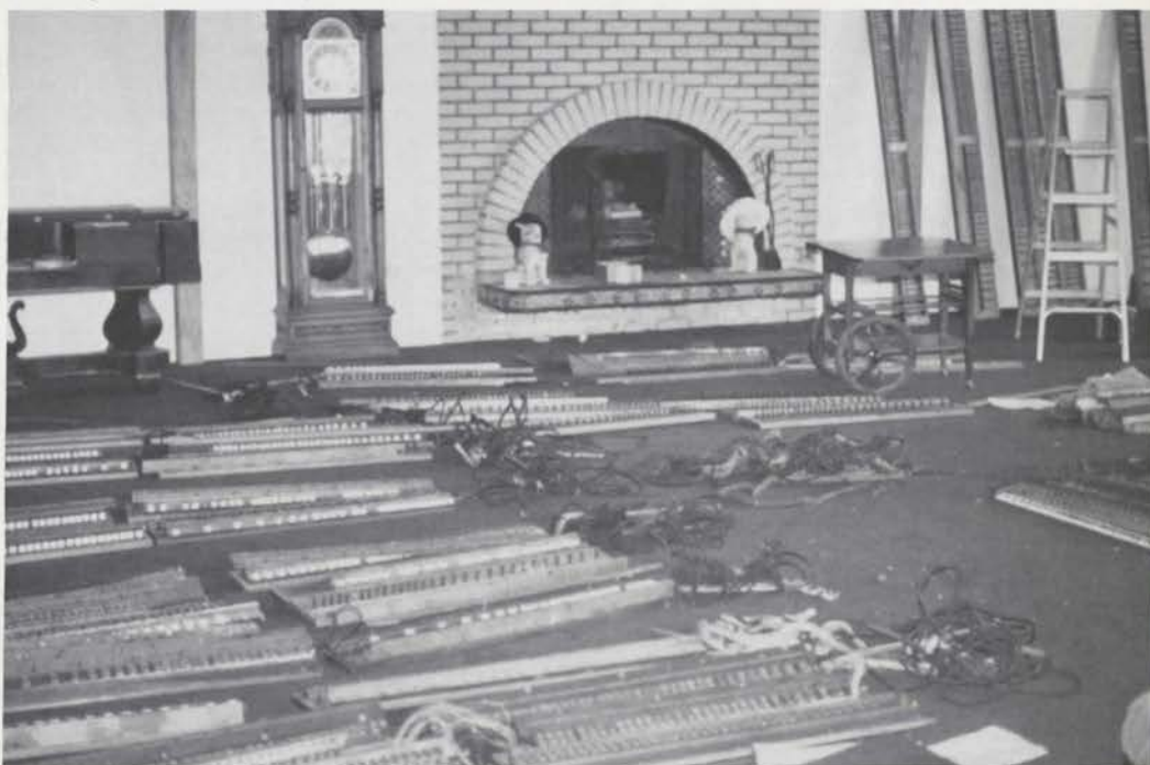
Living room during early stages of rebuilding.
