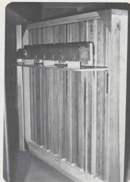
Shutter/chamber access door in open position. (F.R. Gandy photo)
