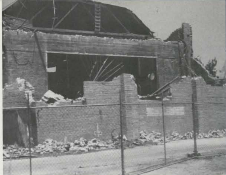
Rear view of the State Theatre, Coalinga, California, showing the stage house collapsed but the concrete proscenium arch still standing. (DeLay photo)
