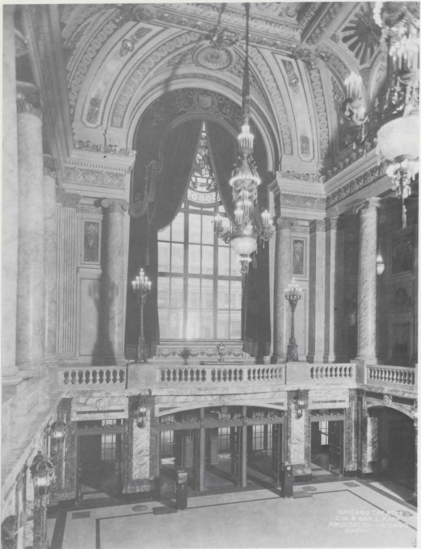
Grand lobby, looking toward main entrance on State Street.
