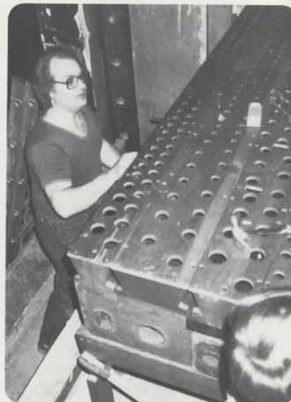
Middletown Paramount crew chief Bob Seeley helps to place solo chest of NYTOS 2/10 Wurlitzer in its chamber.
