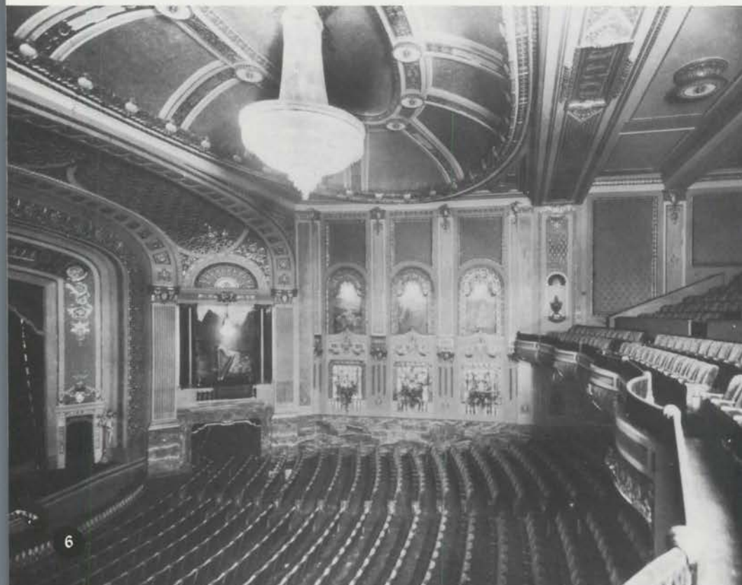
Taken just prior to opening night, this photo shows the massive dome and chandelier, as well as the original inner proscenium which was covered in the 1950s with a Cinemascope screen.
