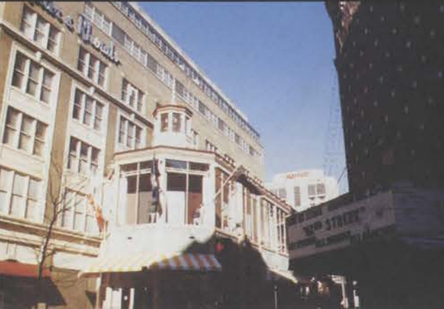
Grace Street entrance to Sixth Street Market Place
