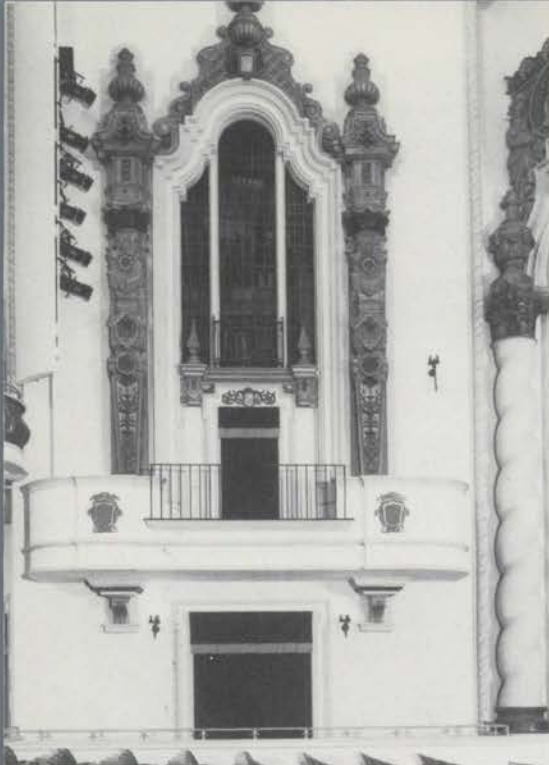
Ornate Spanish grillwork in front of pipe chamber in Saenger Theatre.
