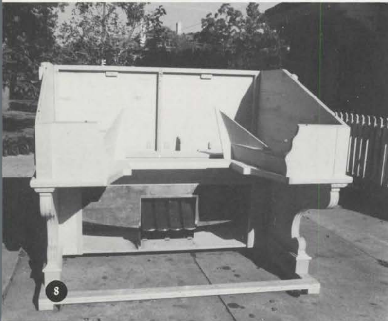
Second phase of console construction. (Note pedal assembly.)
