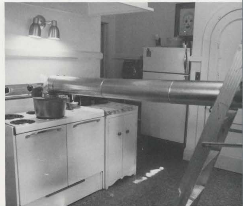
Stop bolsters being steamed inside pipe so they can be bent to fit console.
