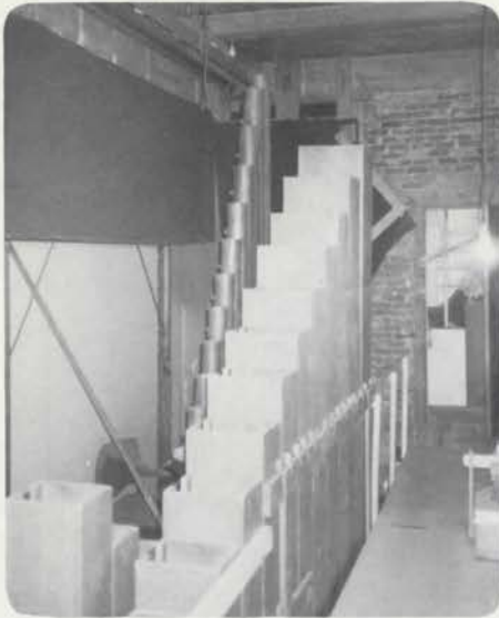
Backstage at the Seattle Neptune Theatre, showing components installed behind the screen and walkway built for access to Solo chamber.
