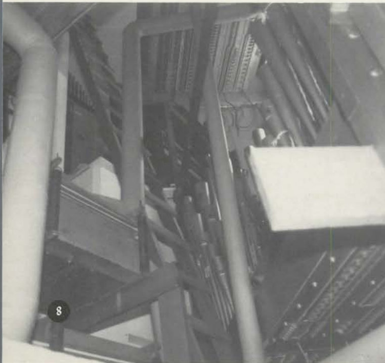
Partial view of Solo chamber showing both levels.
