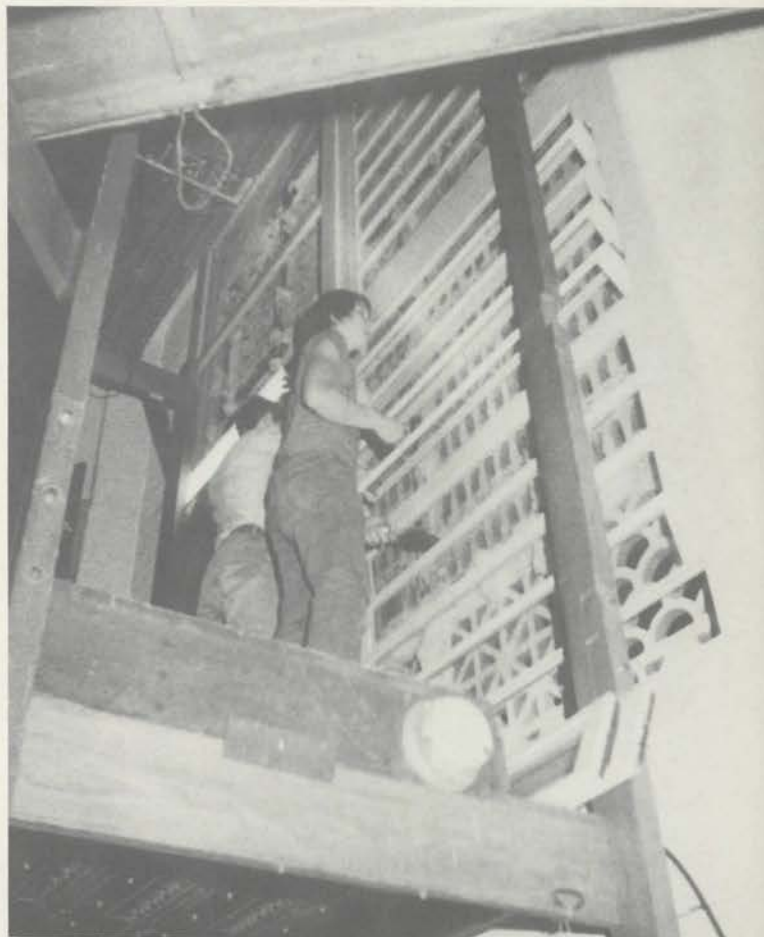
David Junchen and Dan Homberger work on glass swell shades prior to racking pipe-work in Solo chamber.
