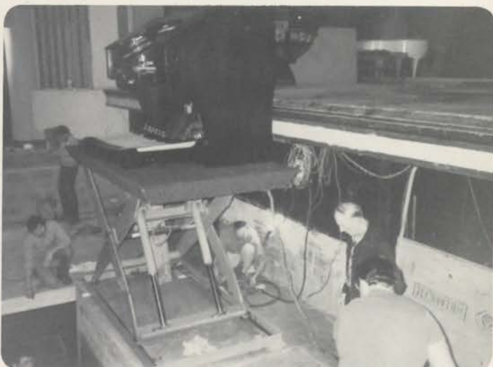
Reconnecting the lift in the Fargo Theatre.
