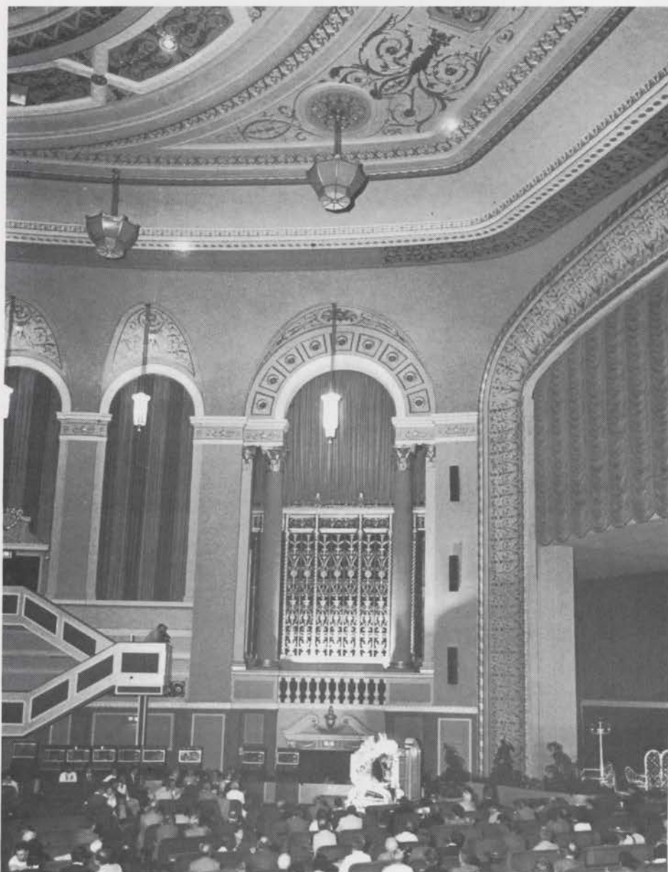
The main auditorium as it is now, with the console in its new position. On the left is one of the new stairways leading from the former balcony to the main floor.
