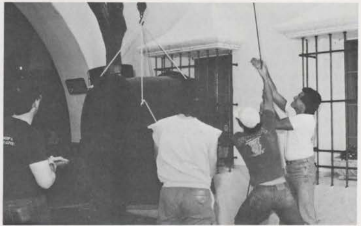
Hoisting the giant blower into the Arlington.
