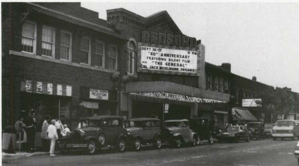
Vintage cars line the street in front of the Redford Theatre.
