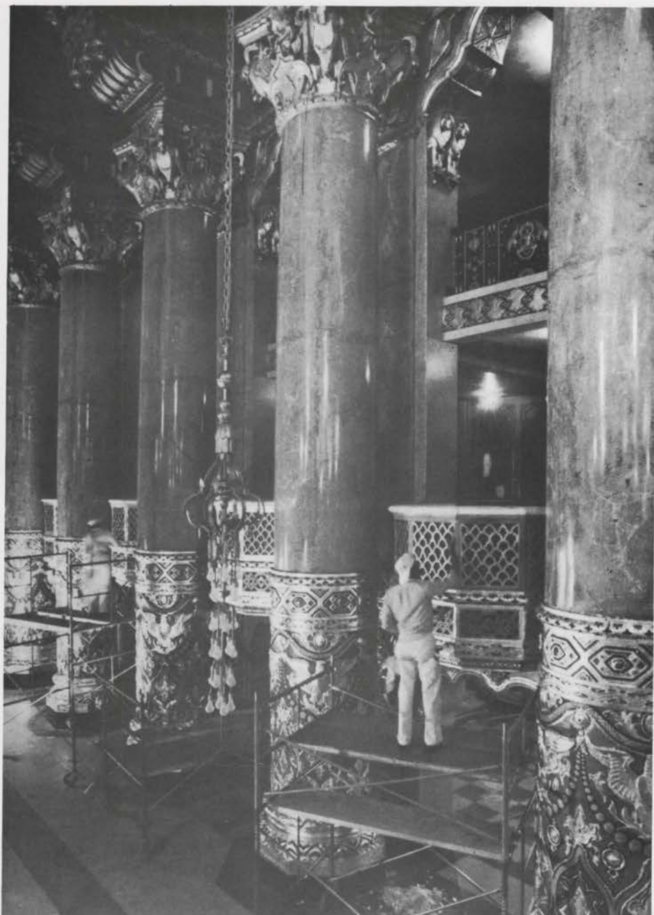
Worker restoring base of column.
