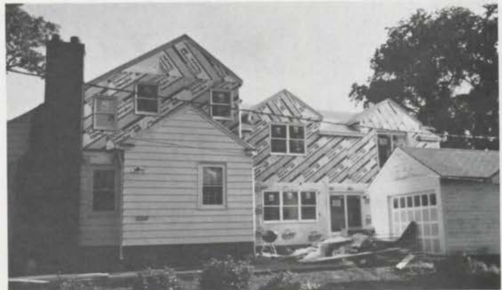
BOB ARNDT'S new music room, which will house his new Arndt "Hope-Jones Unit Orchestra," is only part of the new construction pictured above. The second story blossomed out larger than the first floor.
