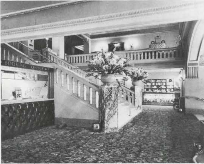
Lobby area of Regent. Fresh flowers daily maintained until closure.
