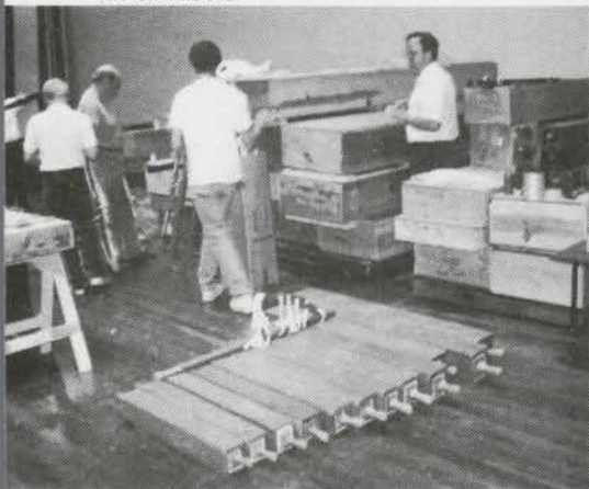
Crates of pipes laid out on the stage ready to go into chambers.
