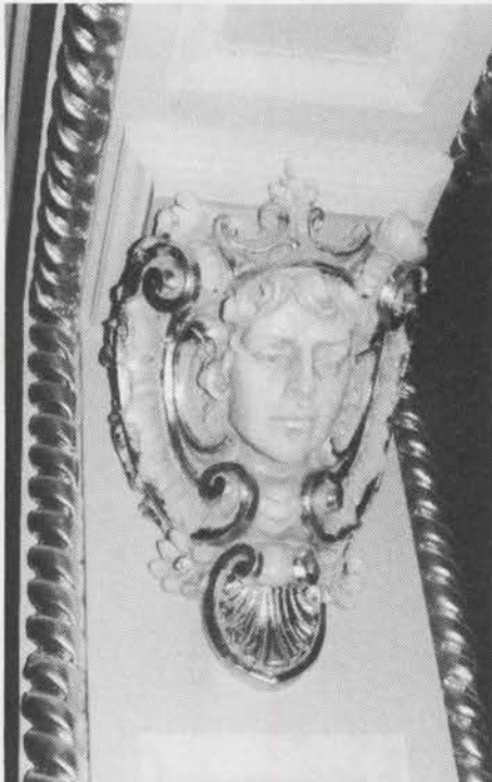
Restored decorative plaster.
