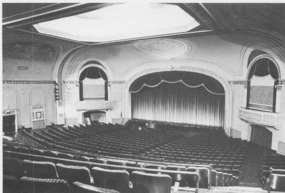
Restored auditorium in Union County Performing Arts Center.
