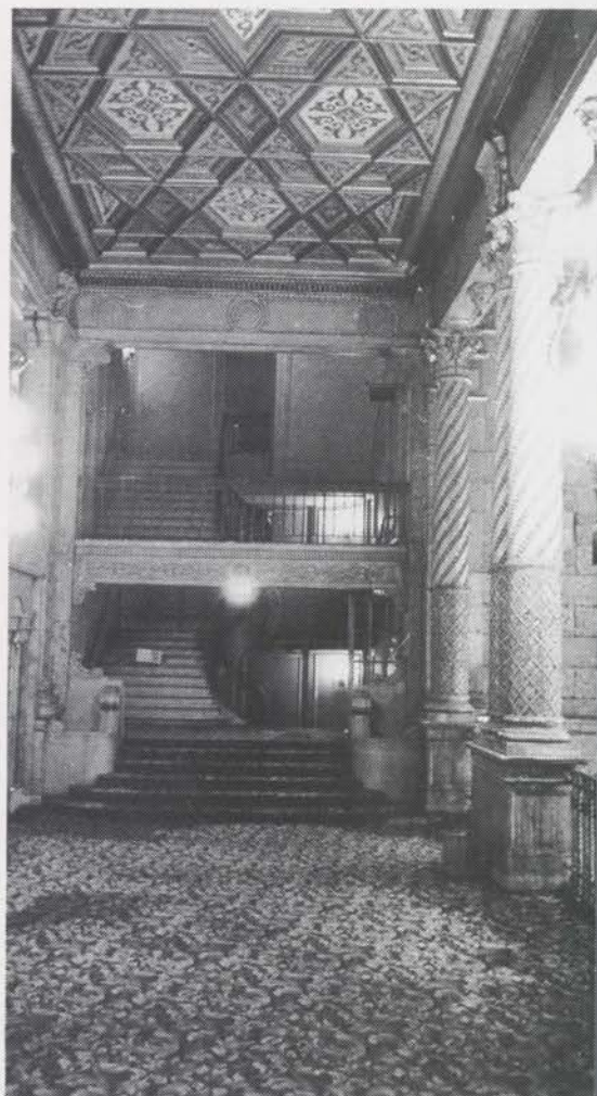
Second floor lobby, 1965.
