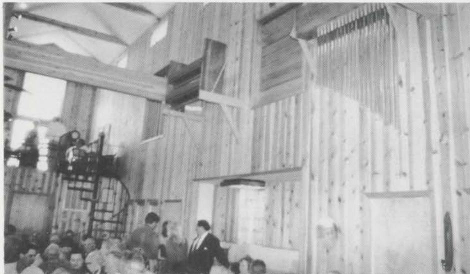
The interior of the Hartzell barn studio.
