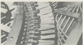
Close-up view of interior of two manual Wurlitzer console showing action pneumatics on top of stop bolster. Note inflated pneumatics. To recover, insert chisel gently under the end of pneumatic, and pry off. Thin leather glued under pneumatics acts as gasket, also allows prying loose without splitting wood ... leather splits instead.
