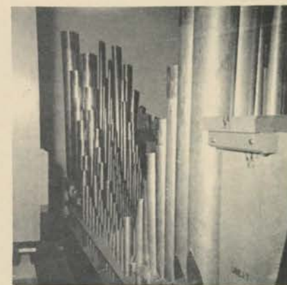
Great chamber principal diapason in foreground, with Gemshorn, Violin Diapason and Tibia Clausa behind.
