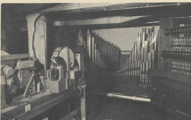
Toy counter on left, harp on right, with pipework in background, Joseph basement.
