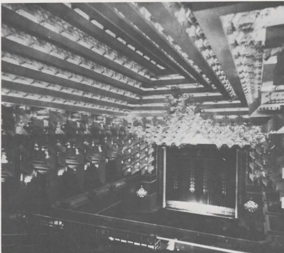
BURLEY GRIFFIN'S MASTERPIECE — The Melbourne Capitol in 1924, showing its famous ceiling. Thousands of concealed colored globes reflected on numerous small plaster prisms, operated from back-stage switchboard.
