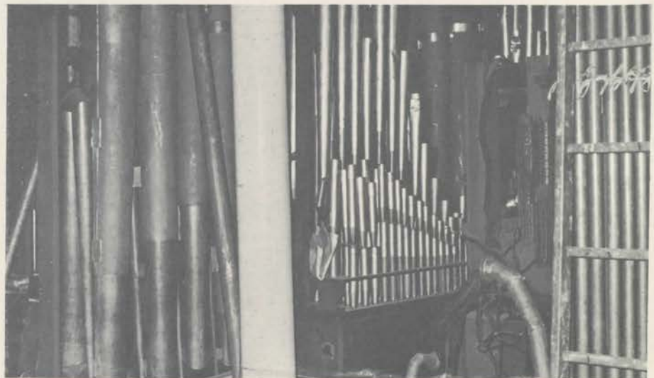
Pipework adjacent to percussion section in ex-Eastman School Wurlitzer. Organ was being dismantled prior to installation in church. -L. Klos Collection
