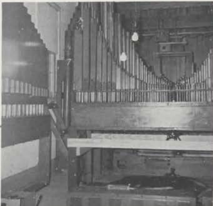
View of Braley Chamber during installation in home.
