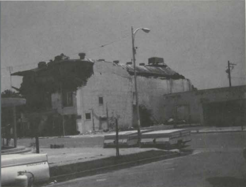
State Theatre, Coalinga, California, after the earthquake.
