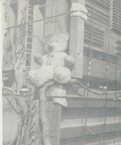
A singed teddy bear guards the switch stacks and relays while they await loading on a truck bound for the Power warehouse for storage. These parts came through the fire almost unscathed because they were located in the cellar — except for water damage.
