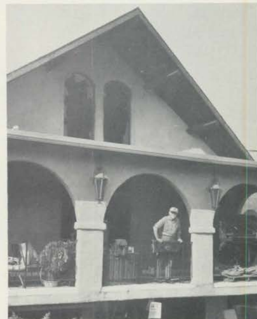
Ray Ledwon, John's dad, awaits the forklift which will lower the console (right niche) to ground level then take it down the steep driveway to the flatbed truck.
