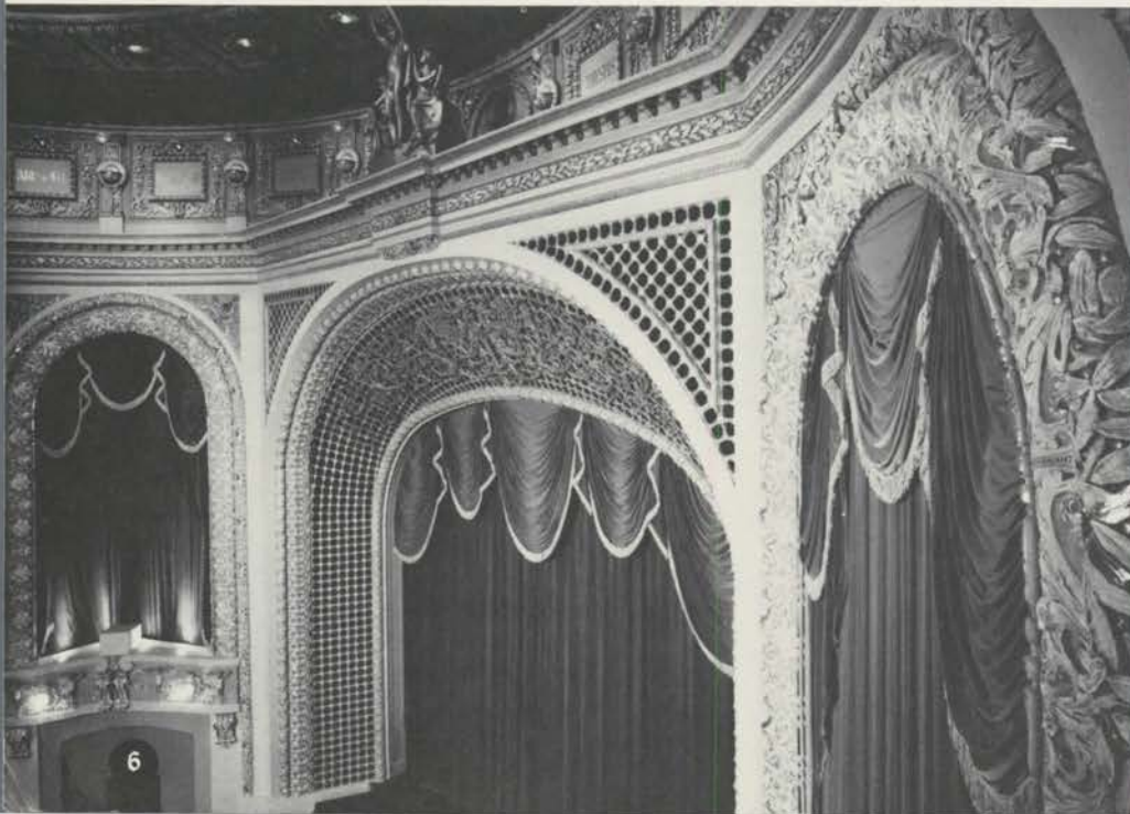
Interior after completion of restoration, a year later. Drapes over organ chambers are acoustically transparent material.
