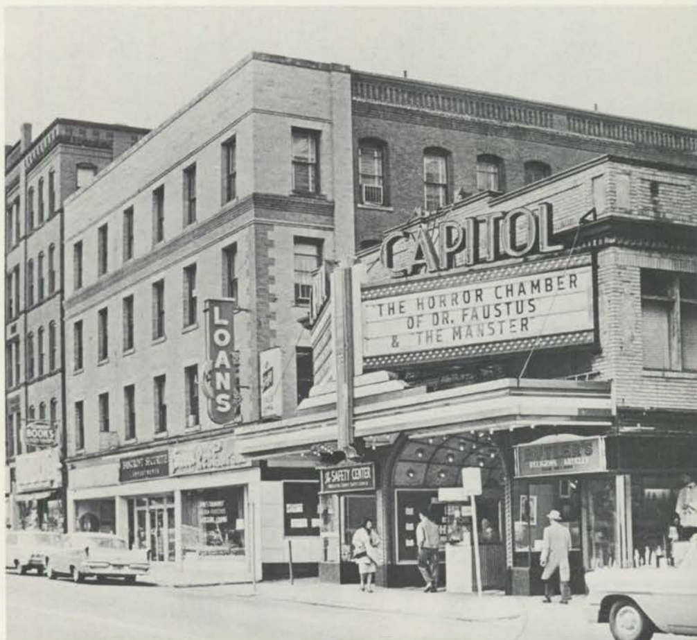
The Capitol Theatre in Worcester, Mass. in June 1962 before renovation. Notice the ornate area above the ticket booth and original marquee and signs which were replaced the following year. (Worcester Gazette Photo)
