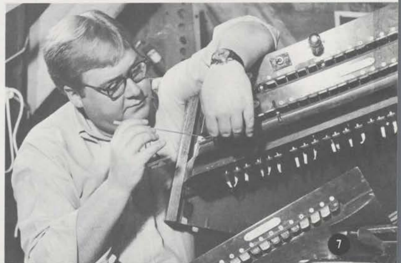
(Below) — Fred Lake installing the solid state relay equipment in the Main Chamber.
