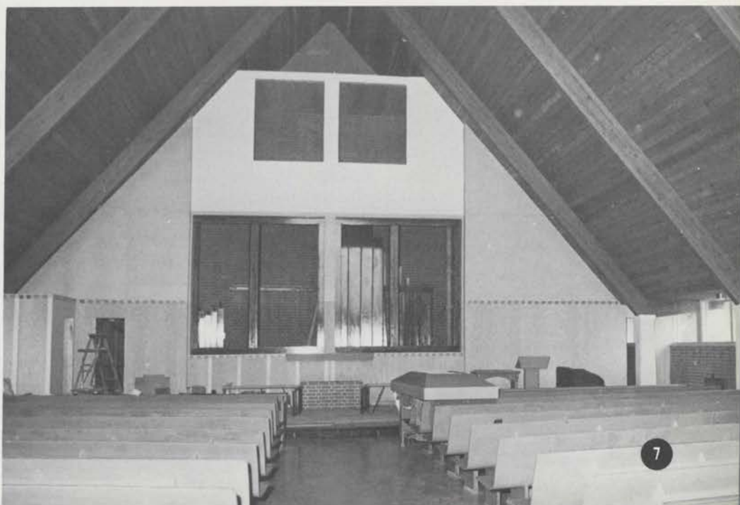
Openings for original Kimball shutters below, and smaller Wurlitzer shutters above for Sunday use.
