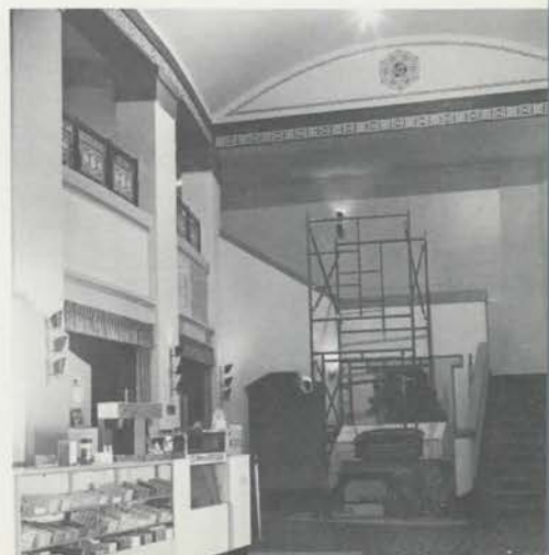
The ongoing restoration in the foyer includes accurate reproductions of the intricate original stenciling, long hidden under layers of paint. Soon, chandeliers from Detroit's Oriental Theatre will be added.
