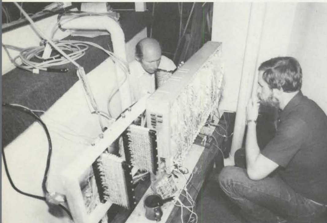
Perkins and Walton wire solid-state relays.
