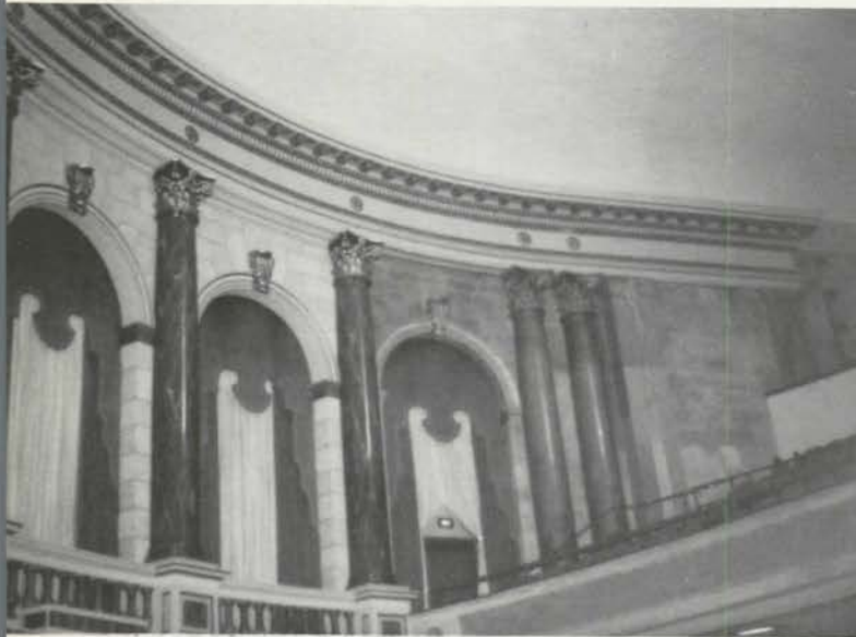
Organ chamber behind left arch. An empty room behind center arch may be used for expansion of the organ. Note unrestored area above right arch.
