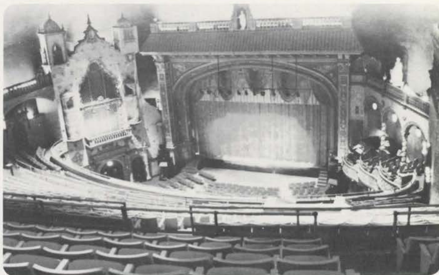
Gusman Cultural Center, Miami, with original 3/15 Wurlitzer, including Piano and 32' Diaphone. Upper right corner of piano visible between chambers on left and proscenium.
