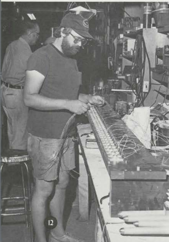
Larry Moen wiring new magnets into an old Wanger in theatre organ.
