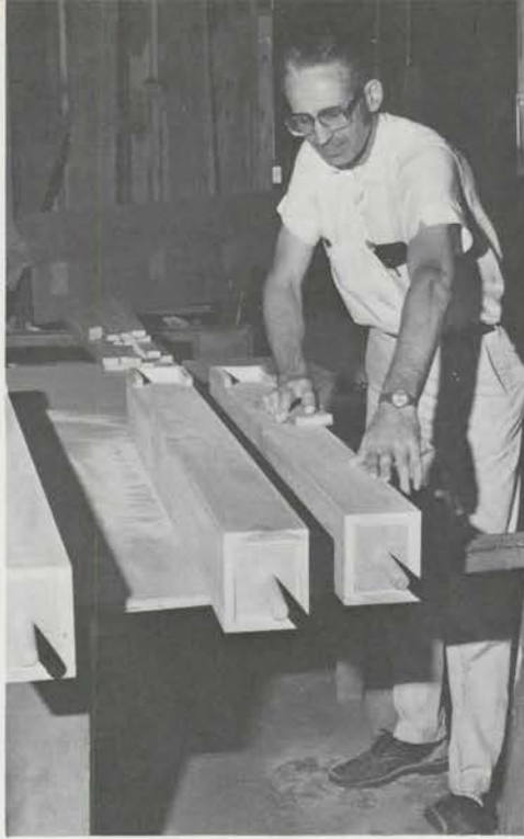
Gerald Schjelderup of Artisan Builders (operating in the Johnson shop) sanding new Tibia pipes.
