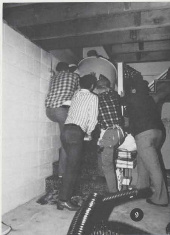
Easing the blower down the stairs into the basement.
