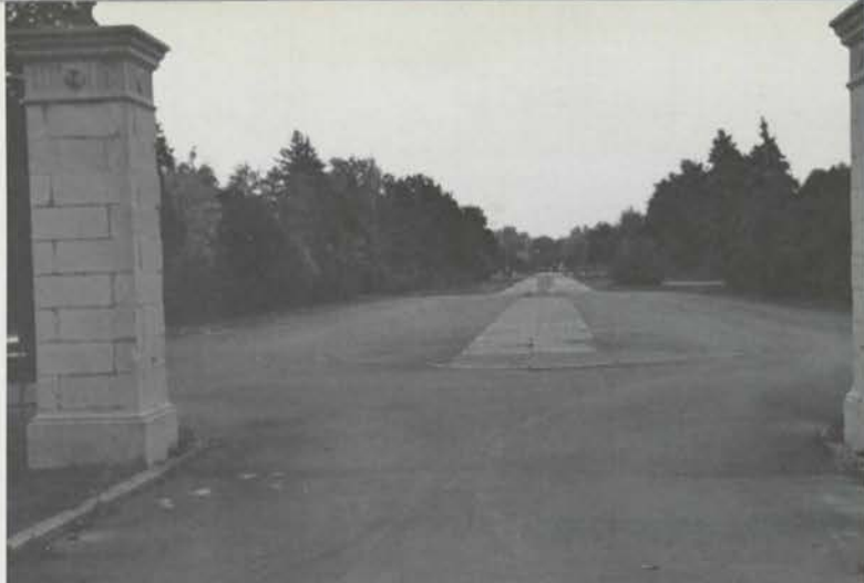
Driveway to plant, looking toward Niagara Falls Boulevard. Area which had shrubs, grass and trees is black-topped. (Klospic)
