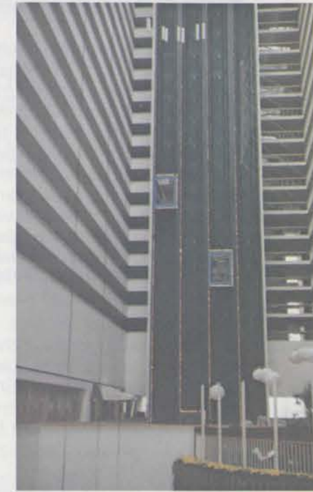
Hyatt Regency — 20-story atrium
