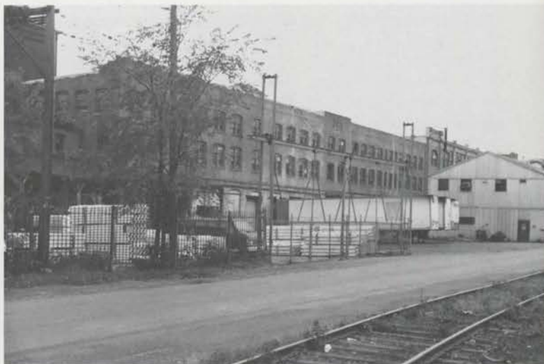
Rear of the factory, showing loading dock area. Railroad spur over which organs were shipped, is shown. (Klospic)
