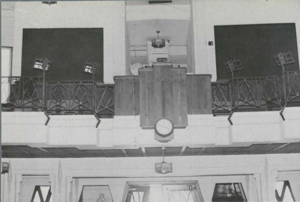
View from altar toward balcony. Solo chamber on left, Main on right. Console is behind wood above clock. Swell shades are covered with sound deadening material.
