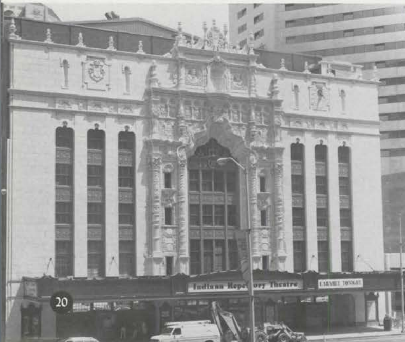
Facade of the Indiana Theatre, across the street from the Hyatt Regency hotel. (CN)
