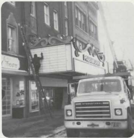
Workmen secure connections from ladders.
