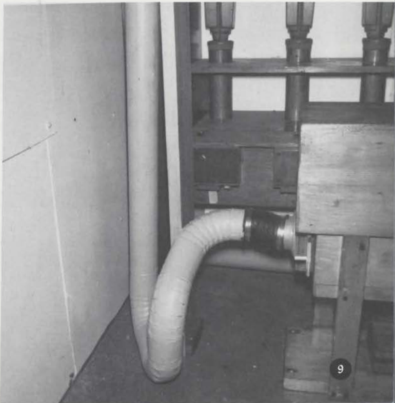
A method of adding elbows on a chamber trem installation.
