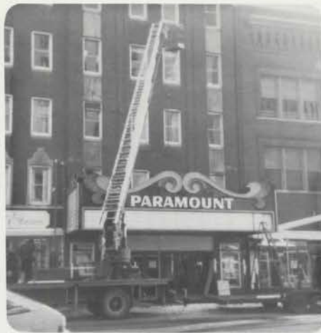
The Cedar Rapids Paramount marquee after installation.
